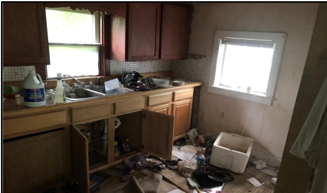
PHOTO: 2 DATE: 6/13/2019 BY: Greg Ross SUBJECT: HA 10: Asbestos-containing adhesive on the ceramic tile backsplash in the kitchen.
