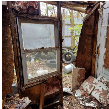
Window With Caulk and Glaze, Room 4
